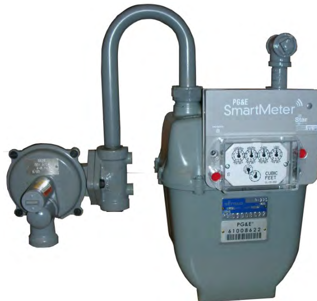
Figure 2-14 Typical Residential Gas Meter Connection
