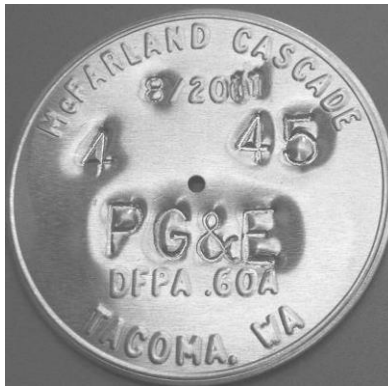
Figure 1. Manufacturer Pole Brand
