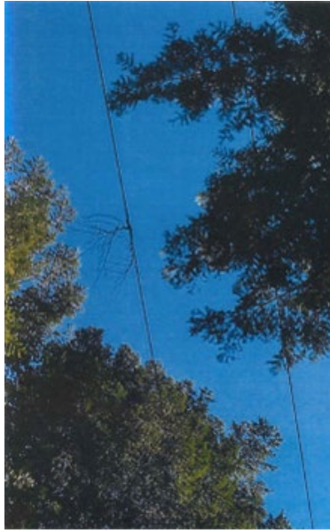
Figure 3-In Nevada City, Nevada County, a tree limb on PG&E conductor. Brunswick 1105 circuit. Address: 14396 GRACIE RD, Nevada City
