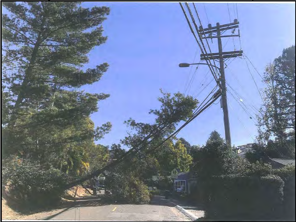
Figure 1: Tree fell onto conductors; Oakland, Alameda County
